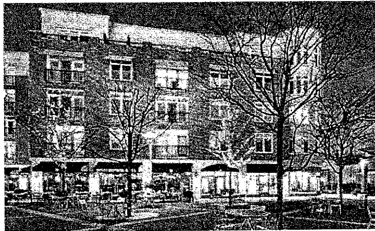
Mixed use development with storefronts providing visual interest. Pedestrian-oriented features encourage pedestrian movement and activity.
